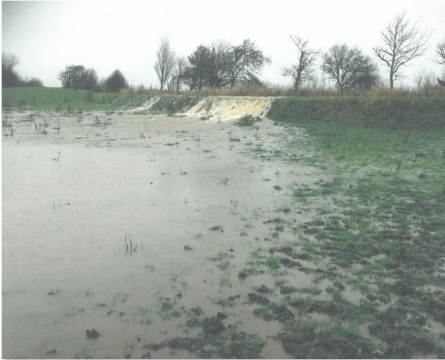
Tributary of Main Drain bank breach, Dec 2015 post Storm's Desmond & Eva
